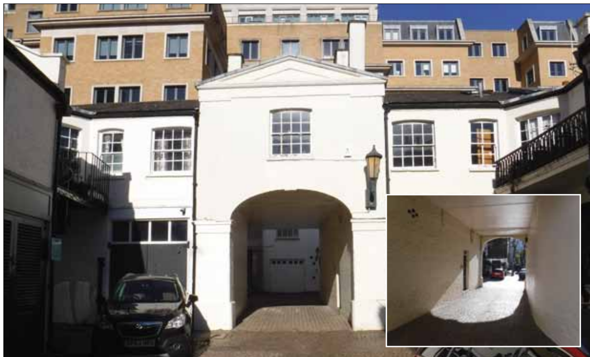
Barrack Yard looking North (Main) and South (Inset).
